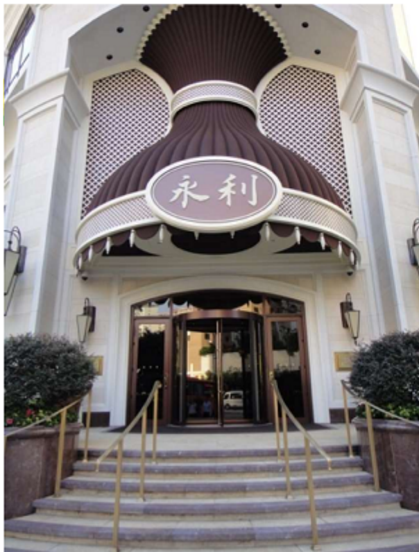
Project: Wynn Casino PPG colour finishing
